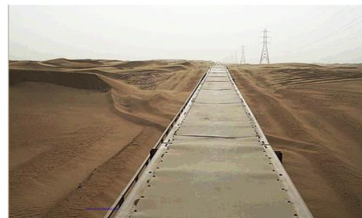
Fig. 2. The longest belt conveyor system (Western Sahara), more than 100 km conveying length (11 flights of up to 11.7 km) [2]
